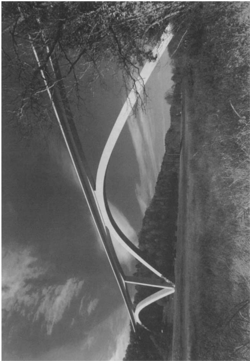
The Natchez Trace Parkway Bridge, located near Franklin Tennessee, was completed in 1994. It earned the 1995 Outstanding Civil Engineering Achievement Award of Merit from the American Society of Civil Engineers. It was the first arch bridge built in the United States from precast concrete segments, as shown in the figure immediately preceding Chapter 1. As such, this bridge combines original technical design with breathtaking aesthetic vision. (Photo courtesy of Figg Engineering Group.)
