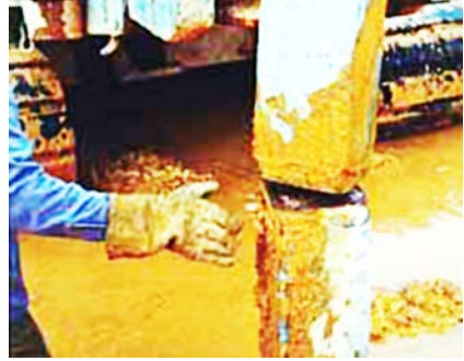
Figure 4.53(b). Insert the new pile to the old.
