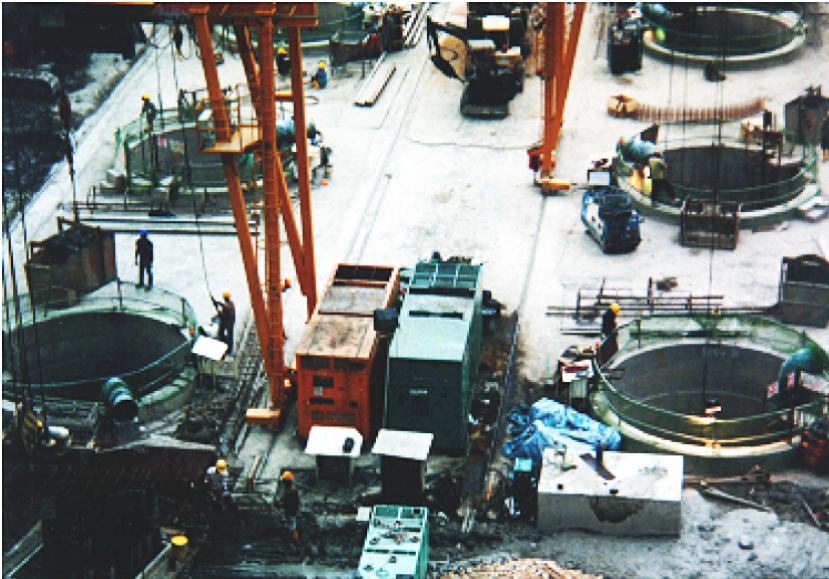
Figure 4.12(c). Two mobile gantry cranes each serving three caissons slide along tracks cast on the concrete floor. Note safety nets on the handrails, artificial ventilators and lighting in each caisson.
