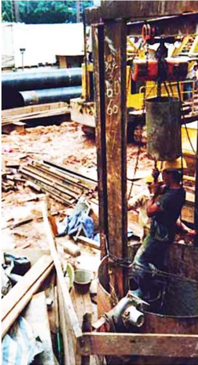
Figure 4.23. Cast caisson to the required height covered with polystyrene for curing.
