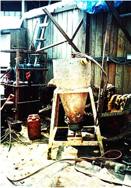
Figure 4.43(a). A hopper to be connected to the top section of the tremie pipe. The hopper acts as a funnel to facilitate the concrete pouring.
