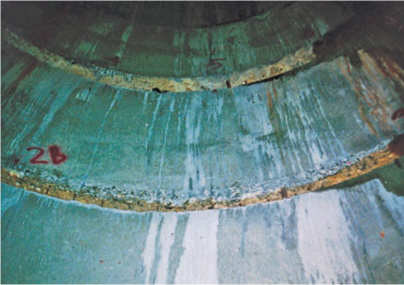
Figure 4.17(a). Completed caisson lining with a gap between each layer.
