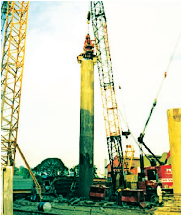
Figure 4.44. The removal of casing after concreting.
