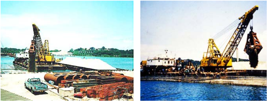
Figure 4.29(c). Filling of sand into a caisson.
