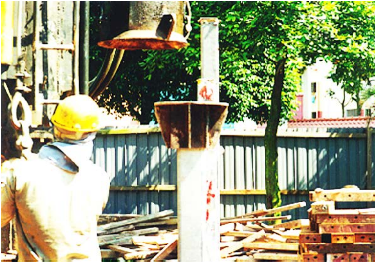
Figure 4.47(b). A mild steel helmet with a 25 mm thick plywood between the helmet and the pile head.
