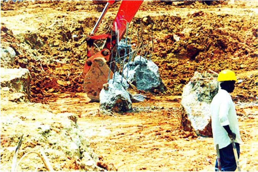
Figure 4.45(a). Excavate to the cut-off level.
