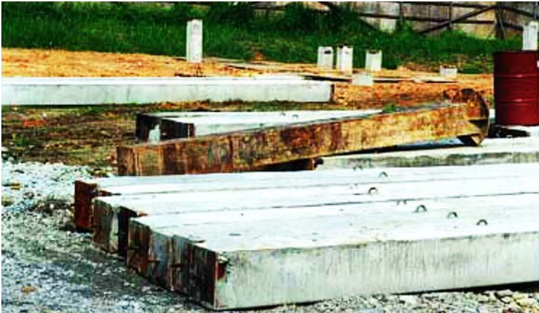
Figure 4.48(a). Pile heads/jointing plates inserted.
