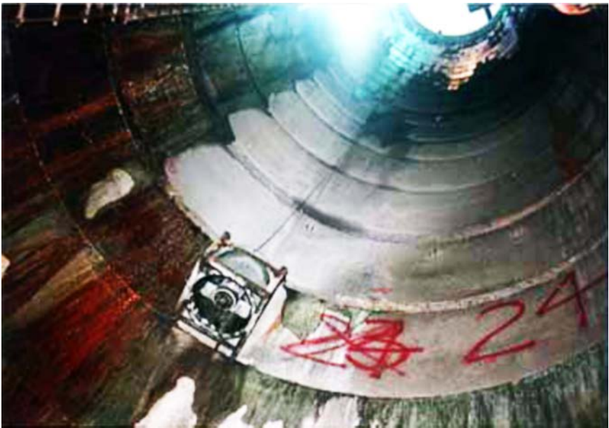
Figure 4.19(b). Provision of a blower.
