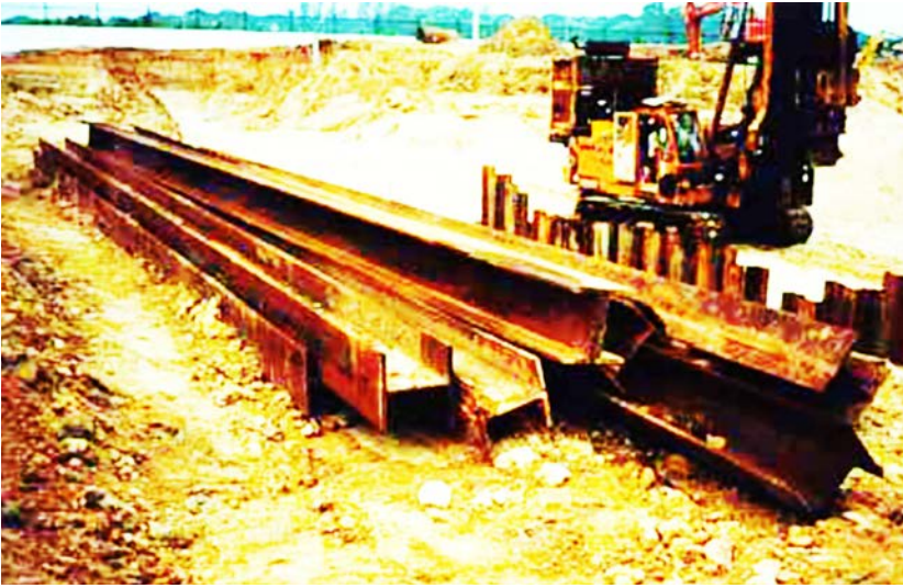
Figure 4.54. Steel preformed H-piles.
