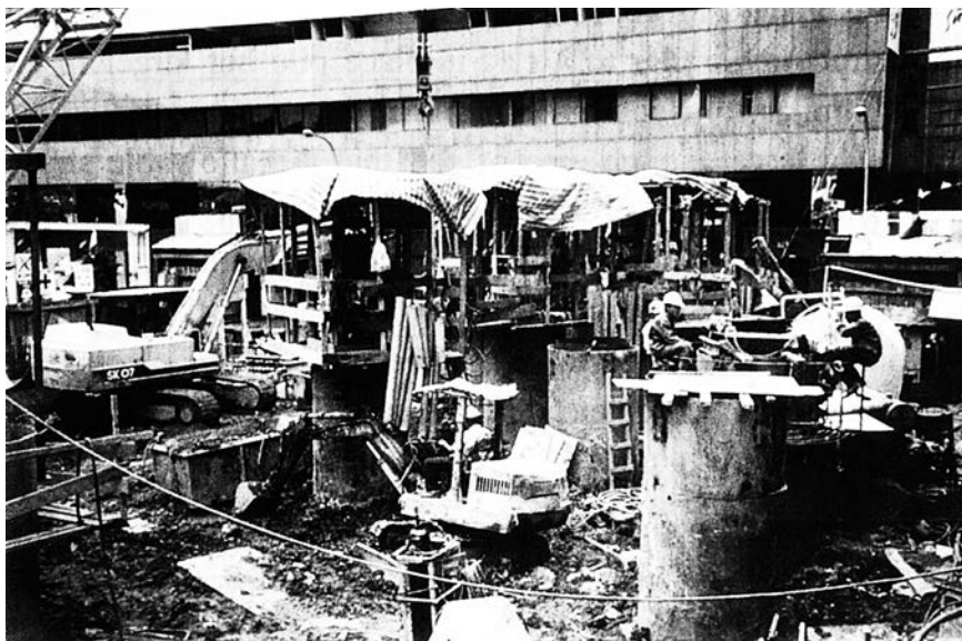
Figure 4.11. Closely spaced hand-dug caissons ( \varnothing \approx 600 mm).
