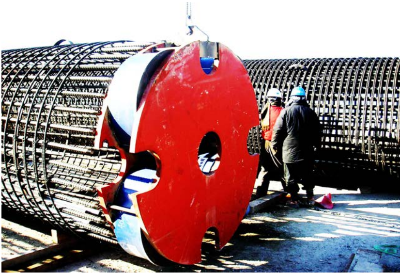
Figure 4.64. Multiple O-cell assembly ready for installation (courtesy: LOADTEST Asia Pte Ltd).
