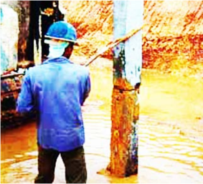
Figure 4.53(c). Align the new pile using a steel fork.
