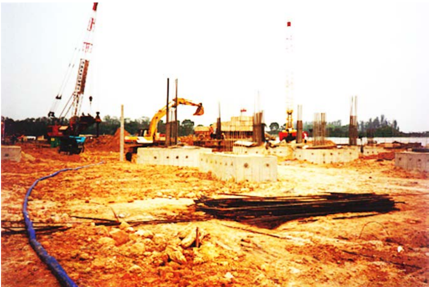
Figure 4.45(d). Construct formwork and cast the pile cap.
