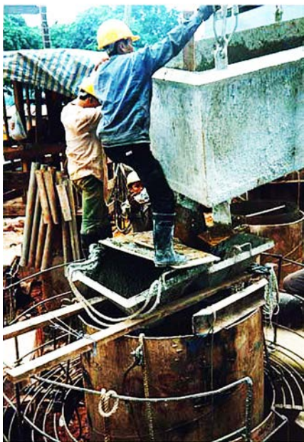
Figure 4.25. Concreting through a tremie pipe into a hand-dug caisson.
