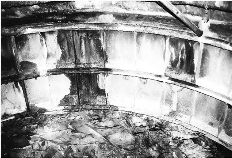
Figure 4.15. Erection of steel ring wall formwork.
