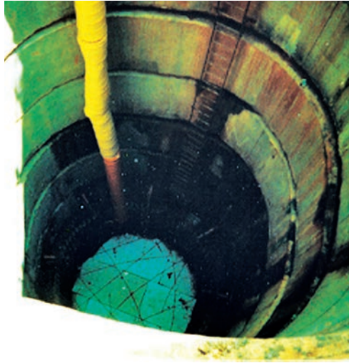
Figure 4.23. Cast caisson to the required height covered with polystyrene for curing.
