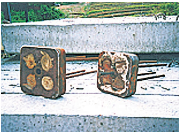
Figure 4.48(b). Pile heads with dowels (male and female).
