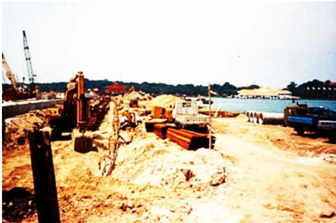
Figure 4.29(d). Caissons filled with sand forming the base of a road link.
