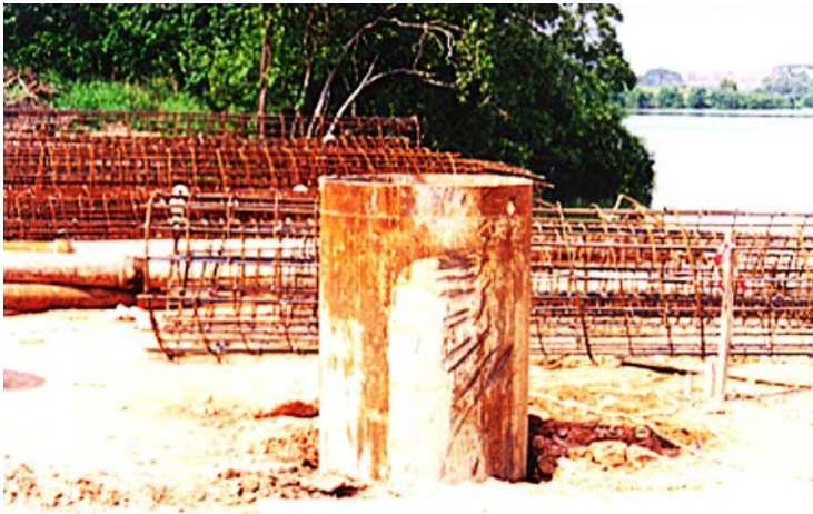
Figure 4.32(b). Protruded steel casing for safety reasons.
