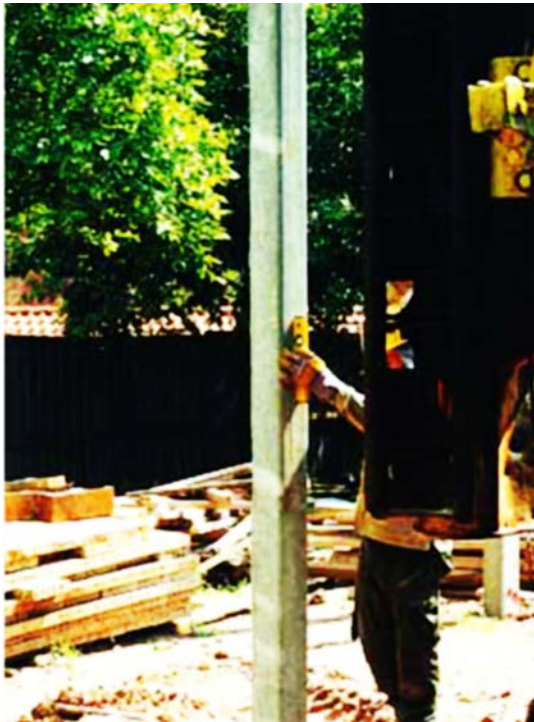
Figure 4.50. Guide the verticality using a spirit level and the leader of the rig.
