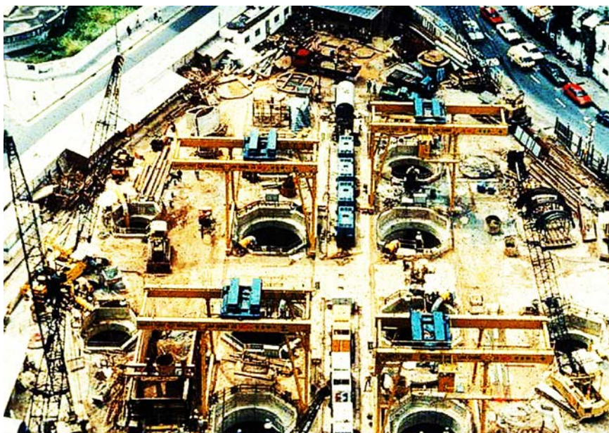
Figure 4.12(a). 12 mechanically-dug caissons ( \varnothing \approx 6 m).
