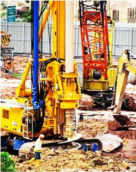
Figure 4.34(a). Removal of soils using an auger.
