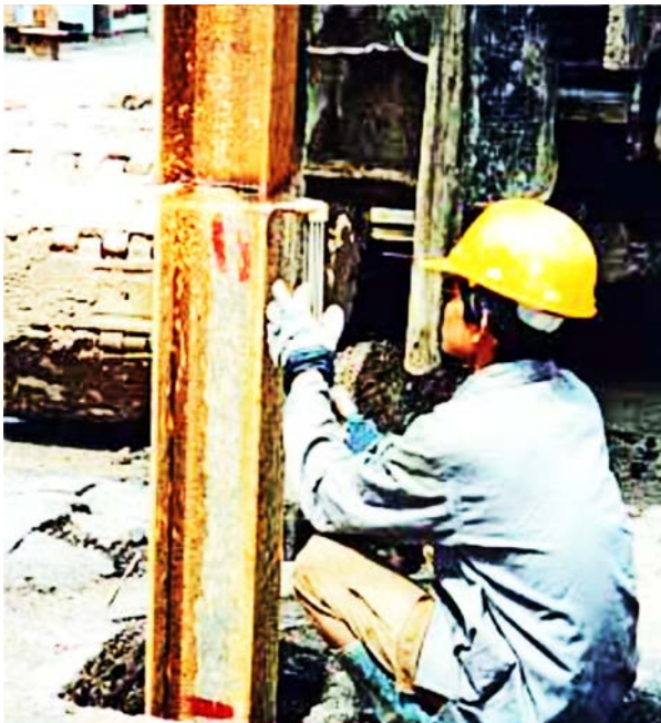
Figure 4.55. Joint welding of steel piles.
