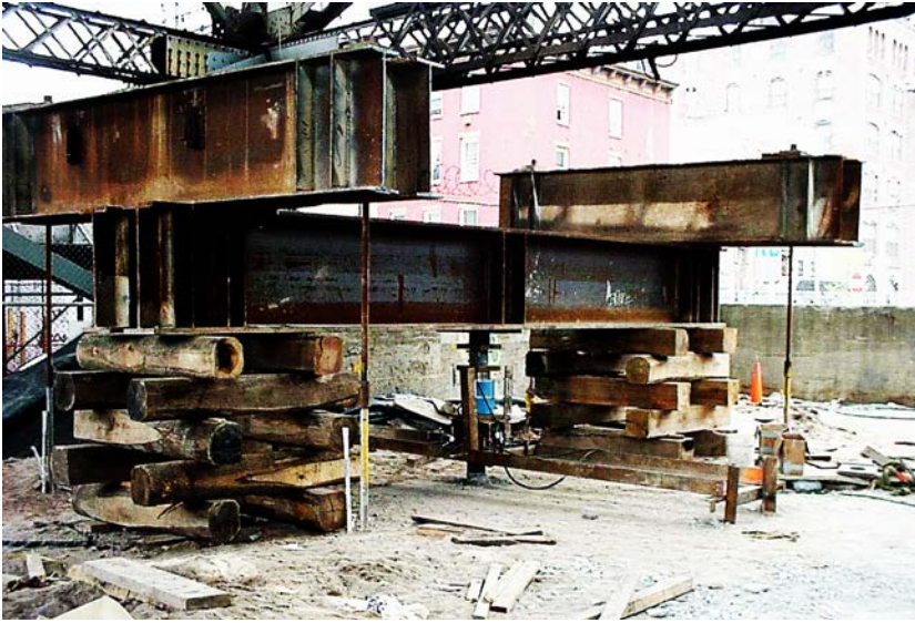
Figure 4.63. An example of pile test using four tension piles (courtesy: Geotechnical Engineering Bureau, State of New York Department of Transportation [37]).
