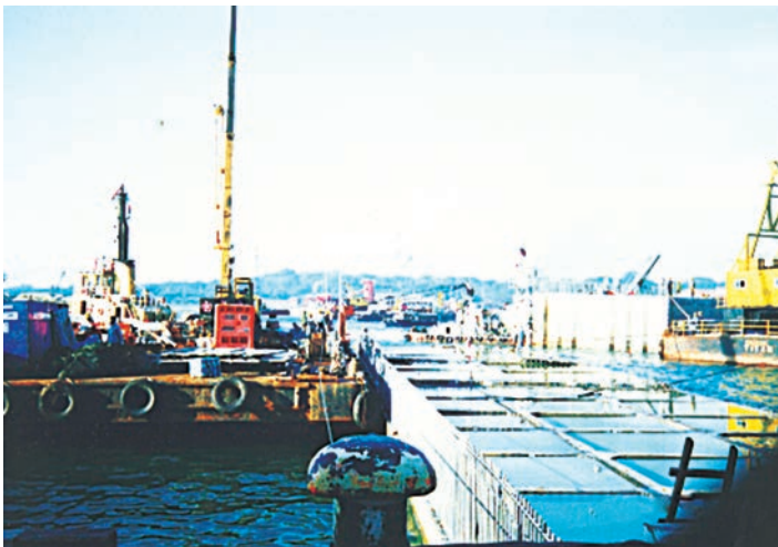
Figure 4.29(b). A tug boat in operation and a submerged caisson filled with water.
