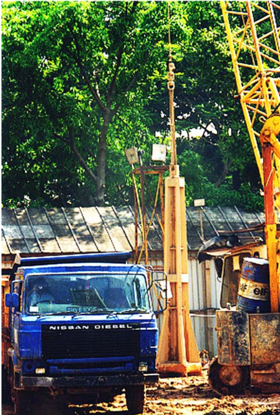
Figure 4.39. Chisels used to break up boulders.
