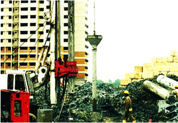
Figure 4.43(c). Tremie pipe hoisted up and down to provide some vibration.
