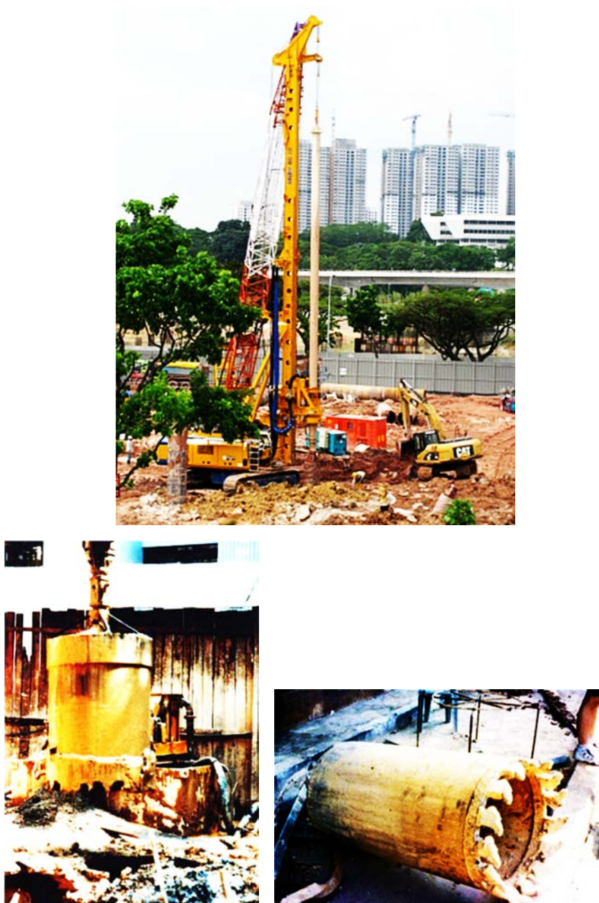
Figure 4.38. A boring core bit for the boring process.
