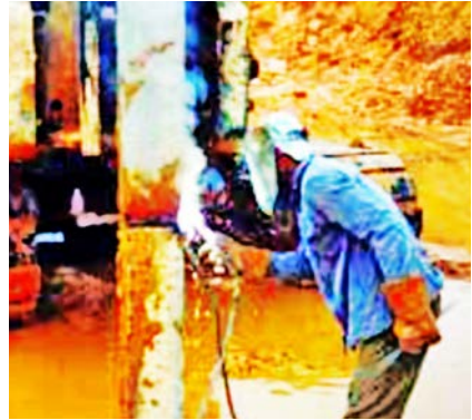
Figure 4.53(d). Weld the joint plate together.
