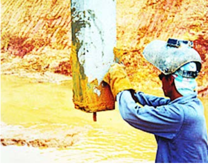
Figure 4.53(a). Lifting of a new pile.
