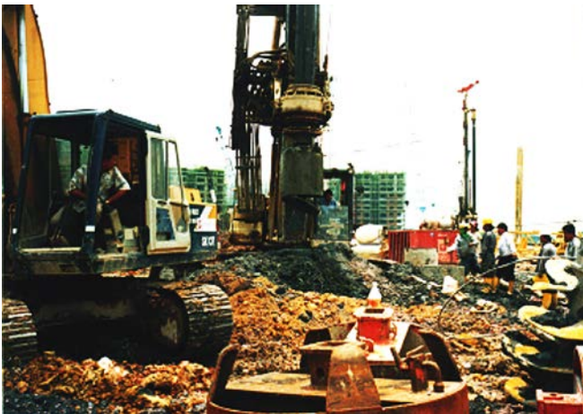
Figure 4.37(b). Shuttle opened to dump waste onto a soil pit.
