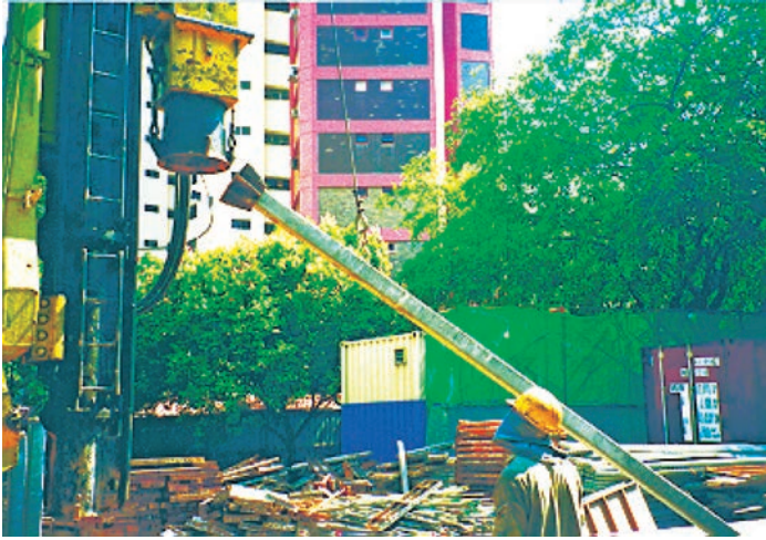
Figure 4.49(a). Hoist up the pile and insert the helmet.
