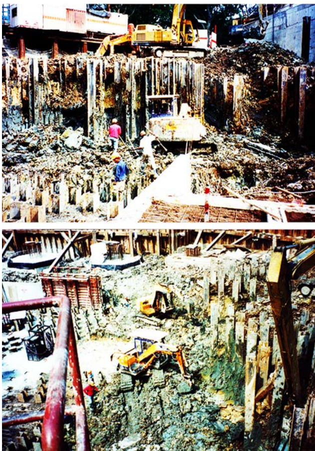
Figure 4.5. Foundation works on marine clay.
