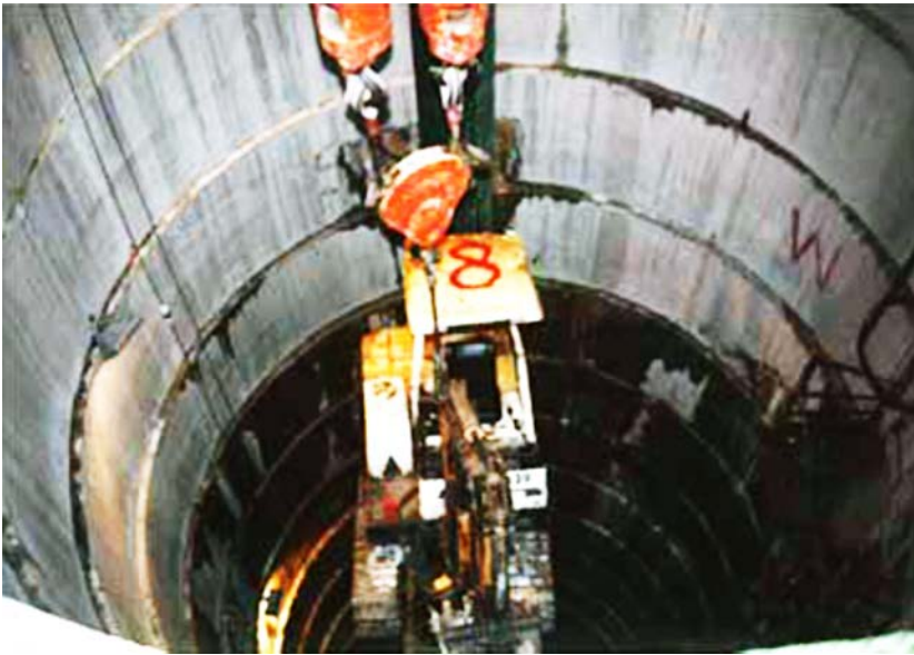
Figure 4.18(a). Lowering a mini excavator using the gantry crane.
