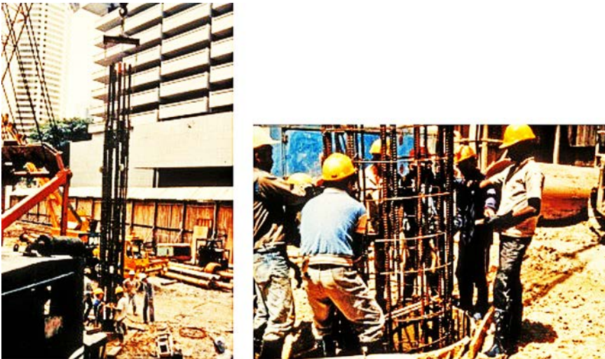
Figure 4.42(a). Insertion of reinforcement cage. Note the 1.2 m lapping between one cage section to another.
