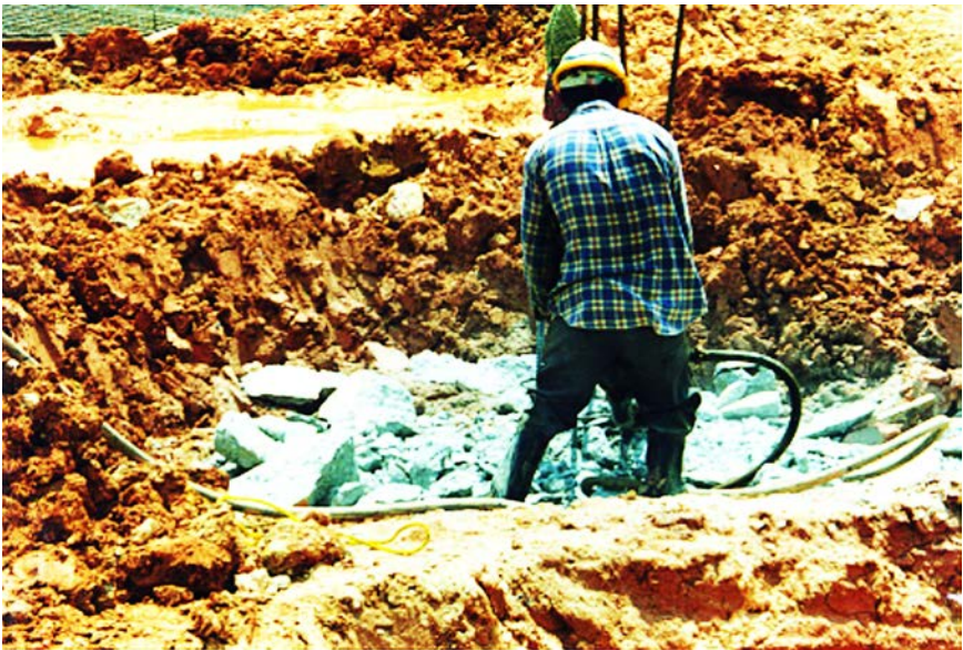
Figure 4.45(b). Hack off the top contaminated excess concrete and expose the reinforcement.
