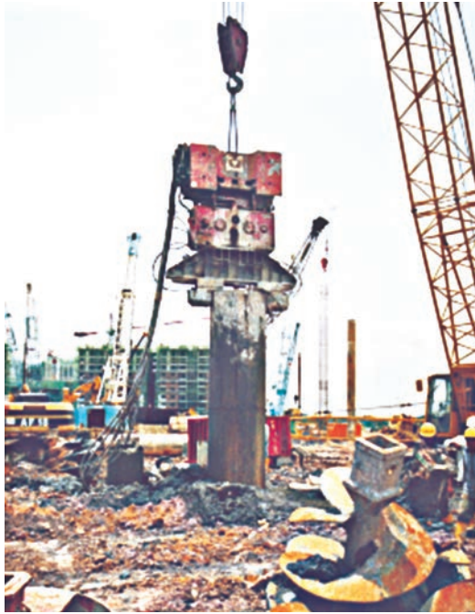
Figure 4.32(a). Insertion of steel casing using vibro hammer operated by the crane operator.
