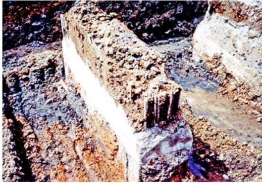
Figure 4.46(b). Example of a barrette pile.
