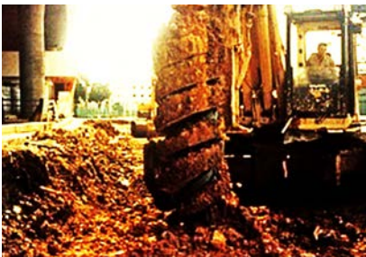
Figure 4.34(b). Augered soil revealing marine clay.
