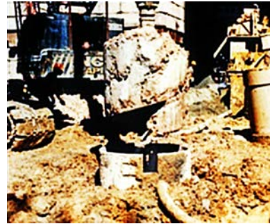
Figure 4.34(a). Removal of soils using an auger.
