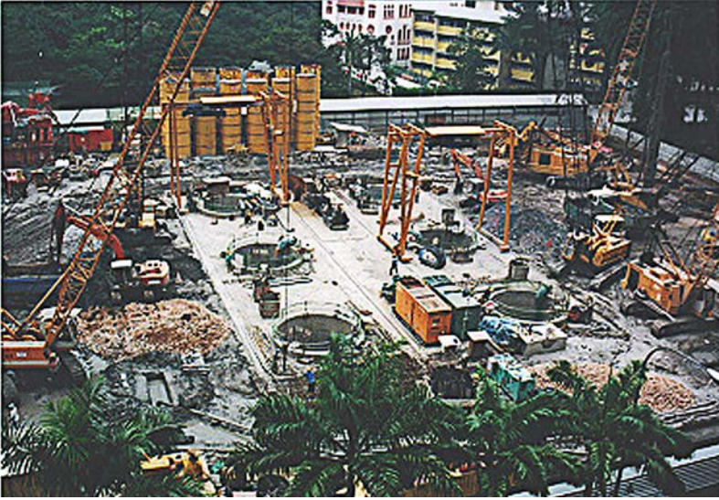
Figure 4.12(b). Construction of six bored caissons ( \varnothing \approx 6 m).
