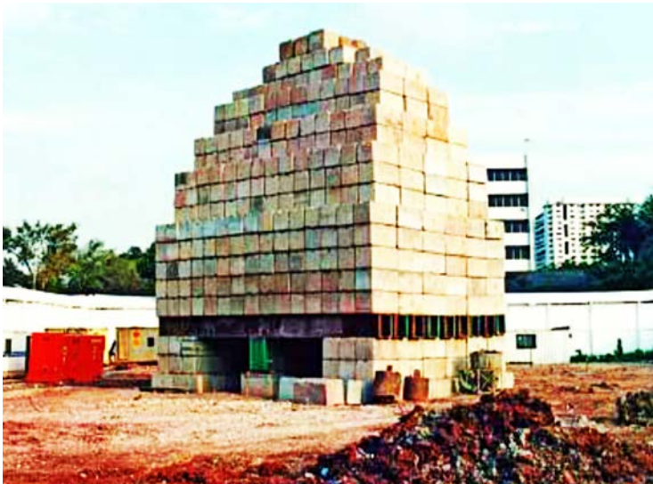
Figure 4.60. Kentledge pile test with stone blocks stacking up on steel channels to act as the weight.
