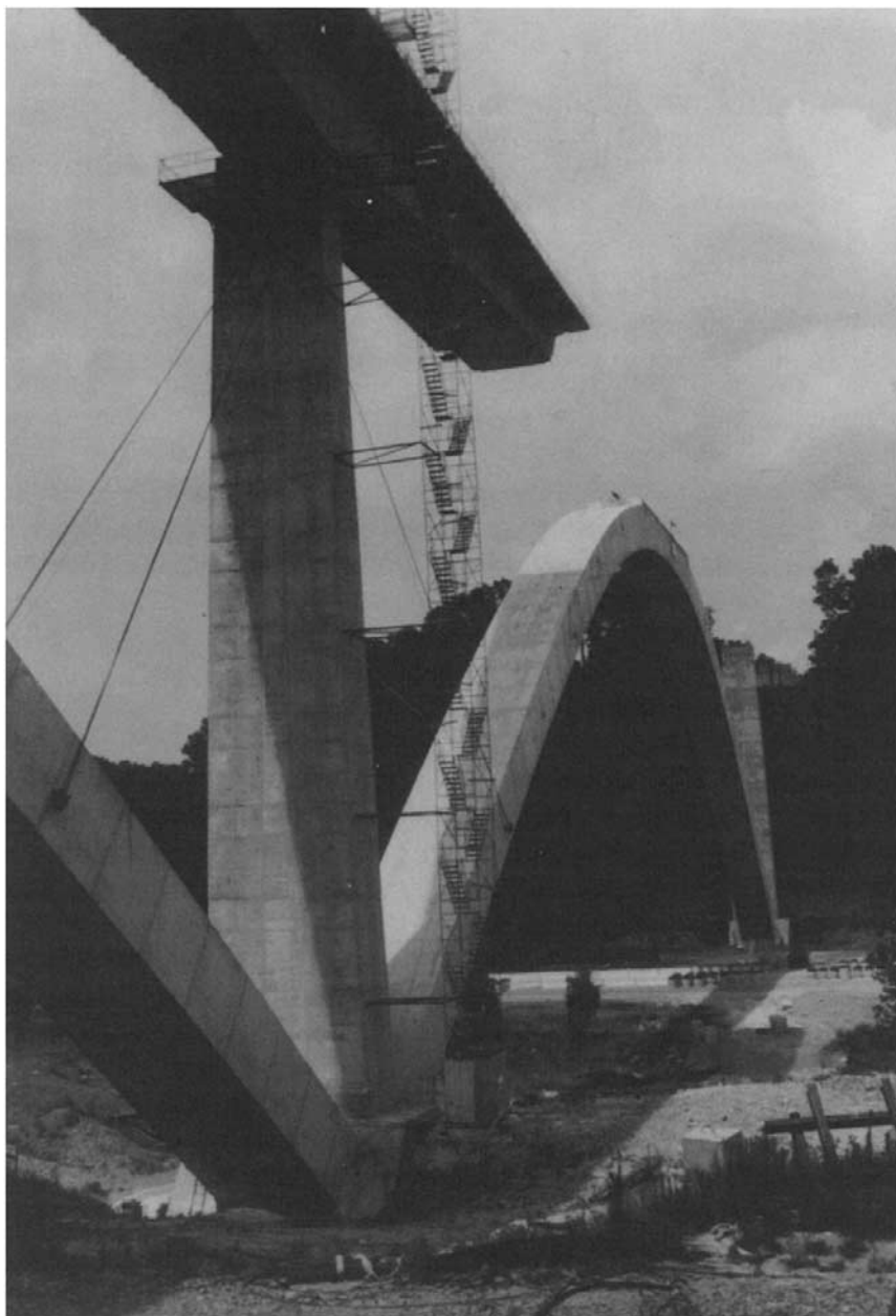
The Natchez Trace Parkway Bridge, here under construction. As noted (cf. Frontispiece), it was the first arch bridge built in the United States from precast concrete segments. Thus, it philosophically is akin to the masonry structures that we show later in the book because it is built up of discrete, blocklike segments. Of course, the designers had the dual advantage of better materials (e.g., the precast, steel-reinforced segments) and of better analysis techniques, the subject which with this book is concerned. (Photo by J. Wayman Williams.)
