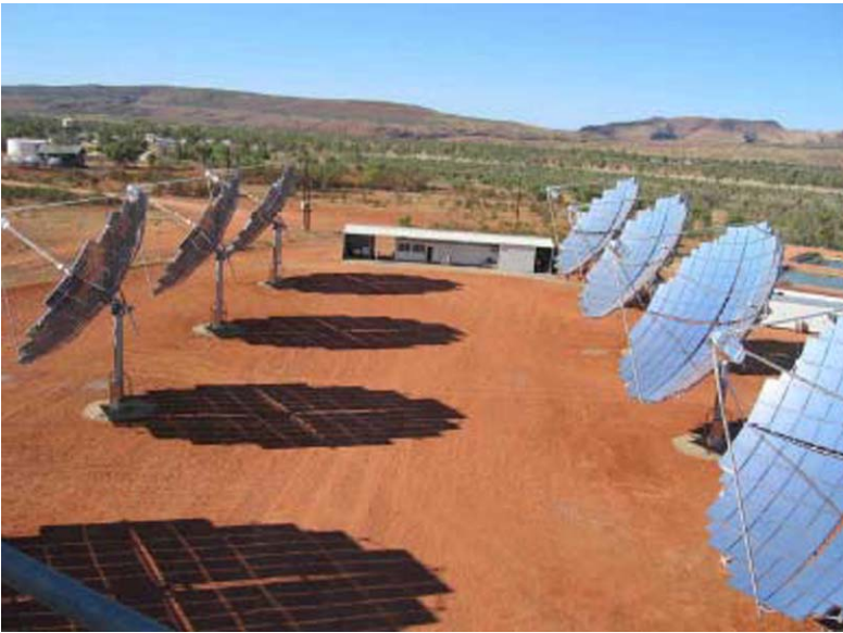
Fig. 2.10. 190 kWp power station by Solar Systems [27]
