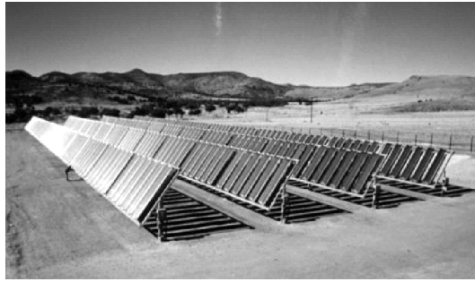
Fig. 1.9. A two-axis tracking 100-kW ENTECH power plant in Texas. System efficiency of up to 14% was demonstrated with this technology at 20 suns: curved Fresnel lenses showed optical efficiency of over 85%. Different cells were used to make the receivers
