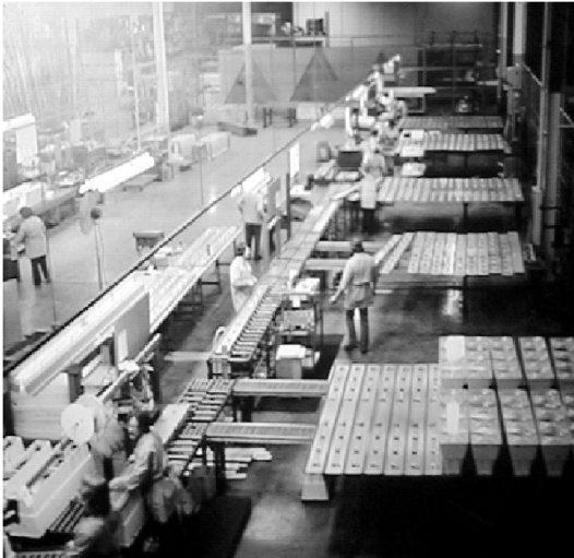
Fig. 1.5. Martin Marietta PV concentrator assembly line built for the SOLERAS project
