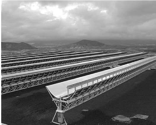
Fig. 1.11. The EUCLIDES demonstration power plant in Tenerife (1998) subsidized by the EU to industrialize the Madrid Prototype (1995). The mirrors were shaped aluminium plates covered with silvered acrylic film which cast 3.2\text{ W/cm}^2 on receivers including SATURN cells. The partners were ITER, BP Solar and UPM
