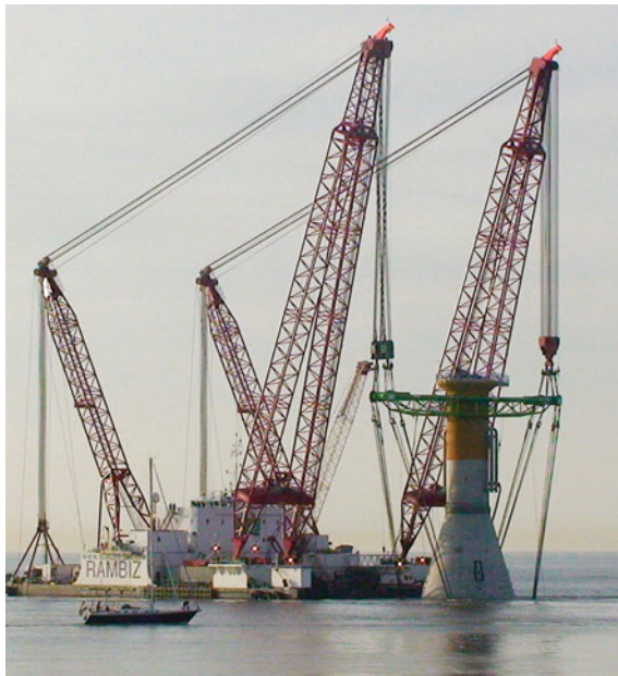
Fig. 2.8 A gravity foundation being installed at Thornton Bank by the heavy-lift vessel Rambiz . Source Luc van Braekel
