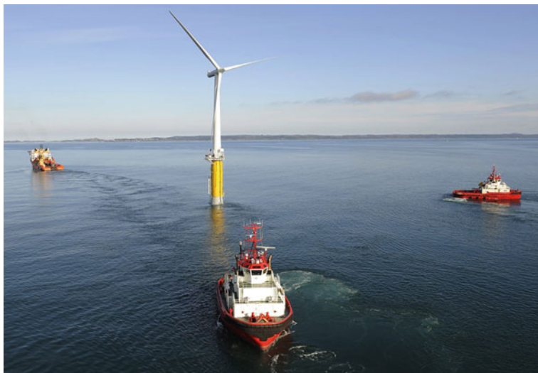
Fig. 2.11 The Hywind turbine being towed offshore. Source Oyvind Hagen/Statoil
