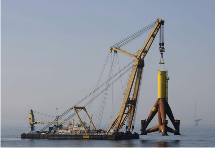
Fig. 2.4 The Taklift 4 placing a tripod foundation at Alpha Ventus. Source Alpha Ventus
