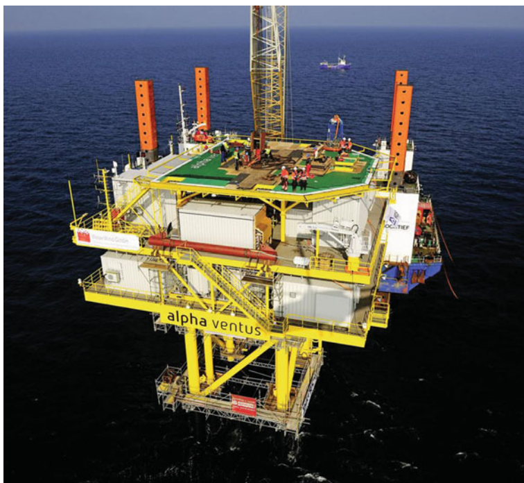
Fig. 2.6 A jacket structure supports the substation at Alpha Ventus. Source Alpha Ventus
