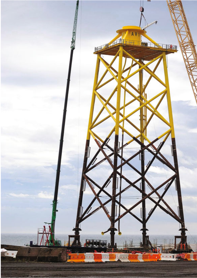
Fig. 2.5 A jacket foundation. Source Alpha Ventus
