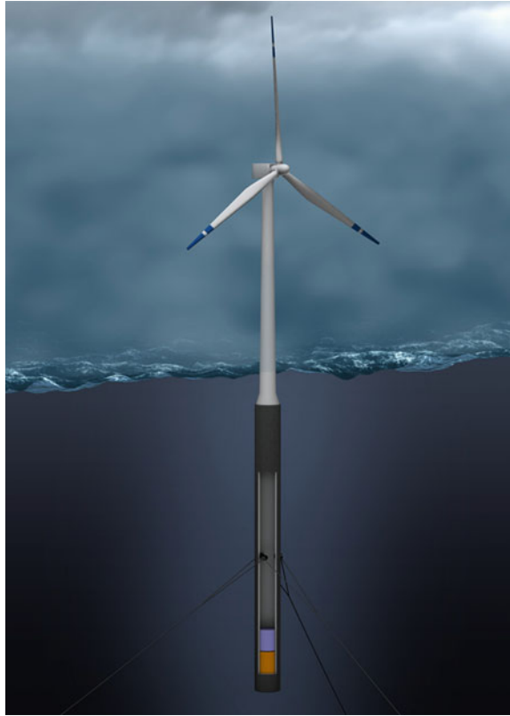
Fig. 2.10 The Hywind turbine and support structure. Source Statoil
