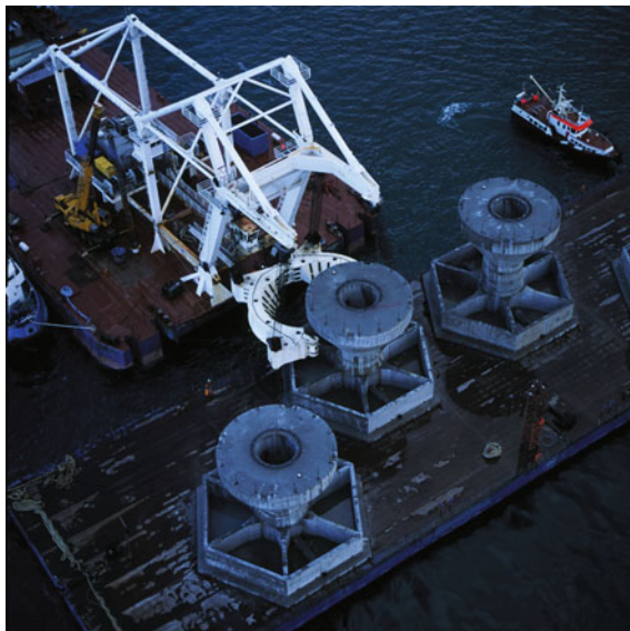
Fig. 2.9 The Eide Barge 5 lifting a gravity foundation from a barge at Nysted. Source DONG Energy
