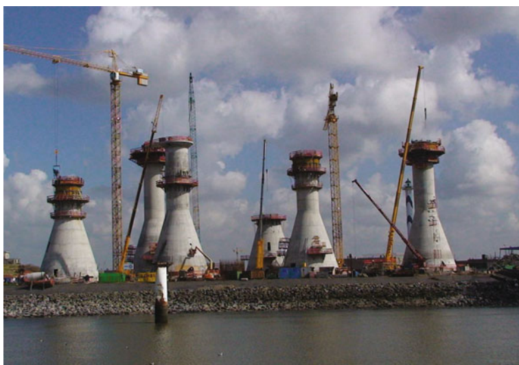
Fig. 2.7 Gravity foundations under construction for Thornton Bank. Source Luc van Braekel
